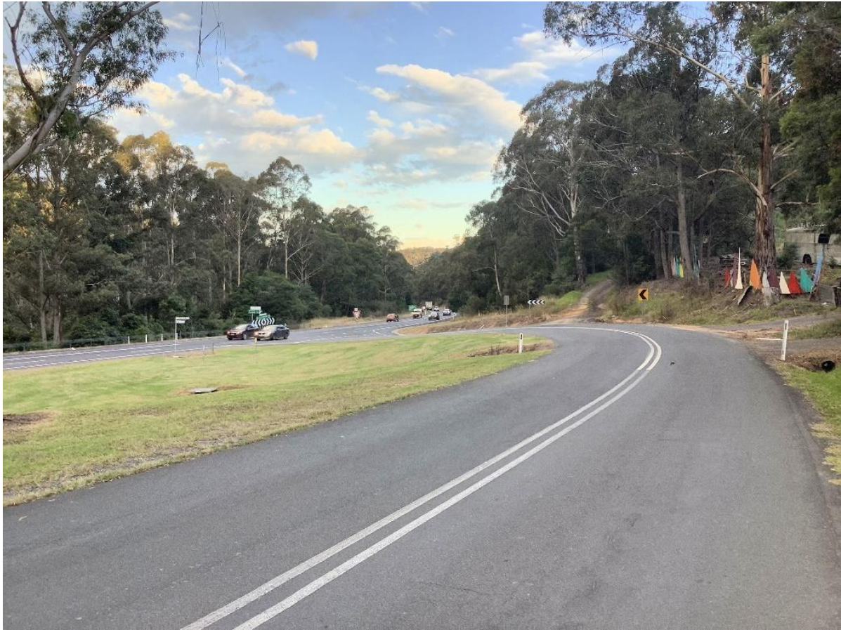
Figure 15 Southern intersection Princes Highway and Wolumla Candelo Road
