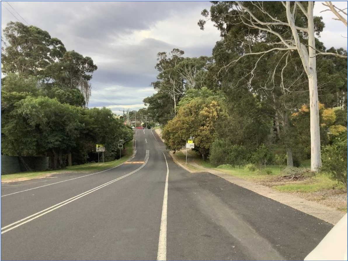
Figure 11 Bega Street view east
